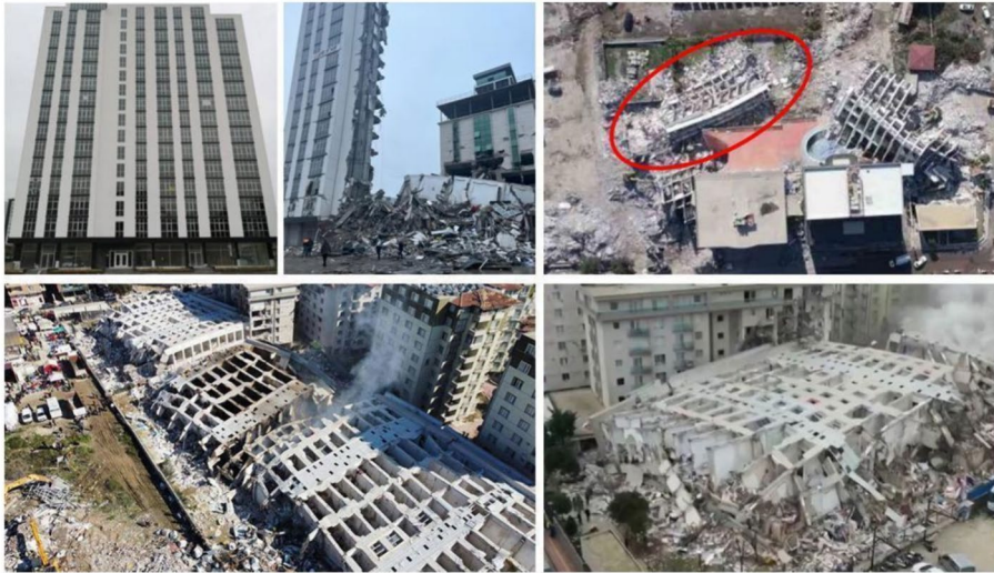
Fig. 11 Post-2000 buildings in İskenderun and in Hatay-Antakya, MCG Tower (above) and Ronisans Residence (below), built in 2009–2011, suffered uprooting collapse, claiming more than 900 lives combined
