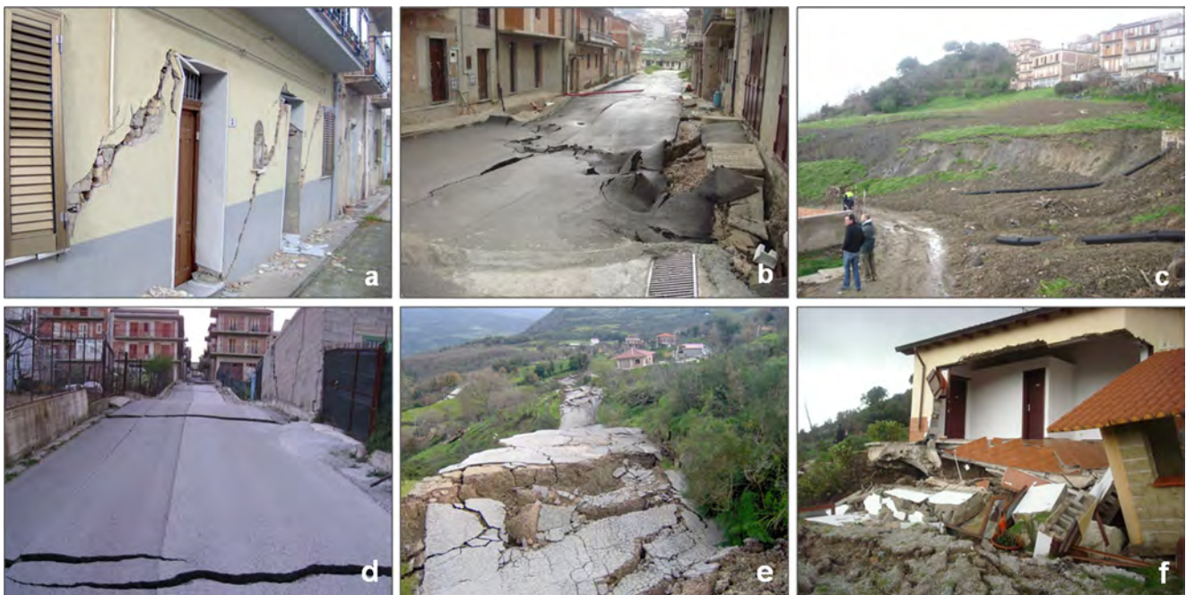
Fig. 3 Example of ground deformations and damage to buildings and structure in the 2010 landslide area. Stazzone quarter: a oriented extensional cracks on building facades and b damaged asphalt road pavement; Riana Quarter: c landslide scarps and d : traction cracks in road pavement; San Benedetto-Porcaro quarters: e country roadway complete failure and f building total collapse (see also Bianchini et al. 2015 for detailed building damage description)
