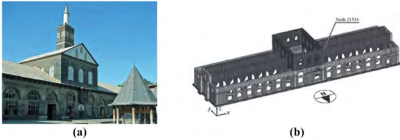
Figure 6. Diyarbakir Grand Mosque: (a) general view and (b) structural numerical model. Figures reproduced from Karaton and Aksoy (2018) with permission, under the terms and conditions of a CC-BY license agreement
