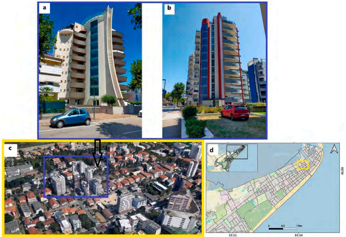
Fig. b.2. An example of the newly constructed high-rise buildings in Lignano (a, b, and c), located at validation stop point number 2. Images in panel a and b are captured by the authors, c map data extracted from Google Earth engine ( https://earthengine.google.com/ ) and d maps data extracted from [26] is available at https://www.openstreetmap.org [91] and is licensed under the Open Data Commons Open Database License (ODbL).
