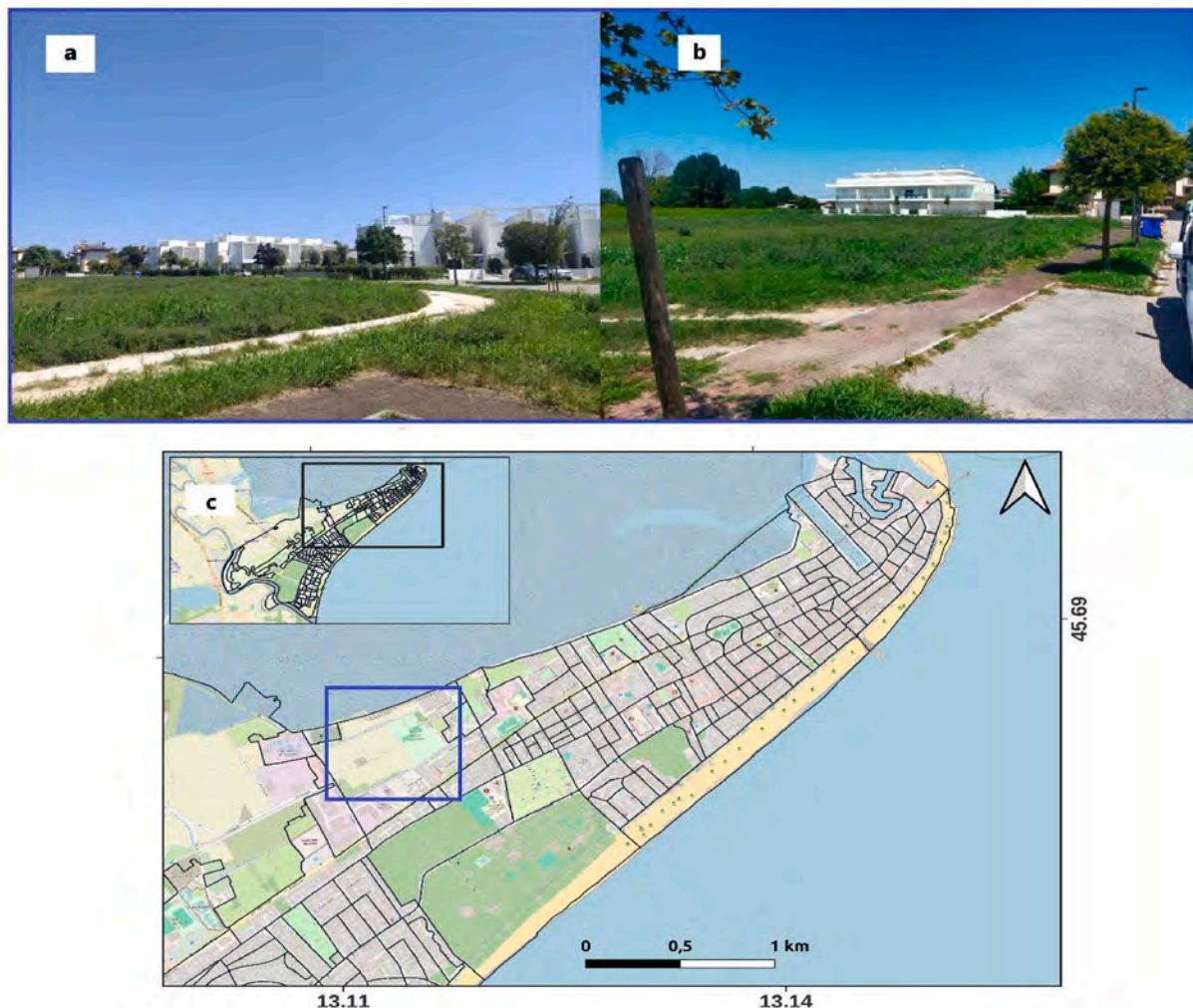
Fig. b.4. An example of the expansion of new building construction in rural areas. The blue polygon represents the census unit, which is comparatively coarser. Images a and b are captured by authors, and the lower map data extracted from [26] is available at https://www.openstreetmap.org [91] and is licensed under the Open Data Commons Open Database License (ODbL).
