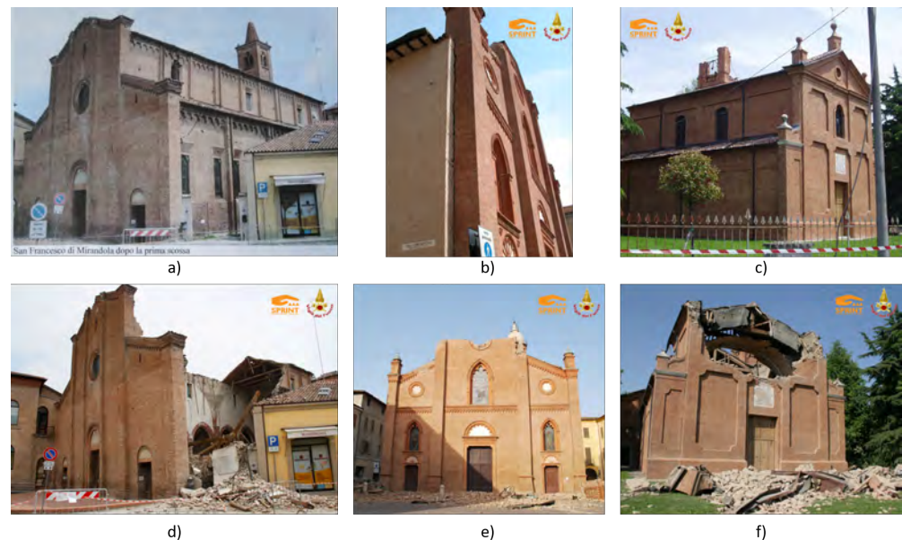
Figure 14. Photos showing the damage of: (a,d) church of San Francesco in Mirandola after the Emilia-Romagna earthquakes of 20 May 2012 (a) and 29 May 2012 (d); (b,e) church of Santa Maria Maggiore in Mirandola after the earthquakes of 20 May 2012 (b) and 29 May 2012 (e); (c,f) church of San Luca in Camurana after the earthquakes of 20 May 2012 (c) and 29 May 2012 (f). The pictures derive from the database of CNVVF-NCP [94], with exception from picture (a) from https://www.italianostramodena.org (accessed on 13 April 2021).
