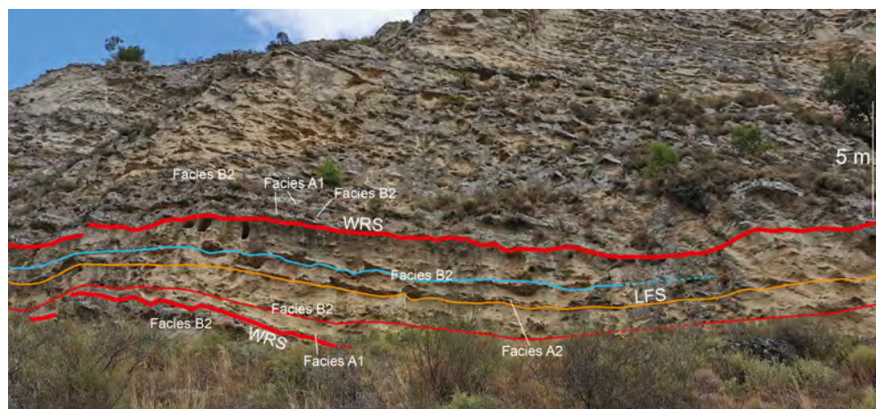
Figure 9. View of the high-frequency sequence documented by the ZNE 2 section (Figures 1D and 5), bounded at the base and at the top by wave-ravinement surfaces (WRS) (see Table 1 for facies code). A local-flooding surface (LFS), close to maximum flooding conditions (see text), is found in the middle of the sequence. A bedset boundary represented by an erosional discontinuity (thin red line) is found in the lower, transgressive part of the sequence, whereas another bedset boundary, represented by a non-depositional discontinuity (thin blue line) is found in the regressive part.
