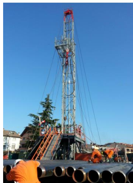
Figure 5. Grado - 2 drilling by direct circulation rotary rig on derrick.
