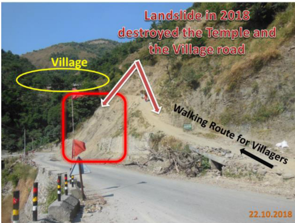
Figure 1. Landslide in 2018 razed the village access road and temple near Amroha.
